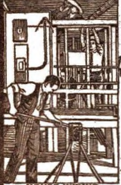
HOUSE WIRING only one of the many branches you "Learn By Doing."
